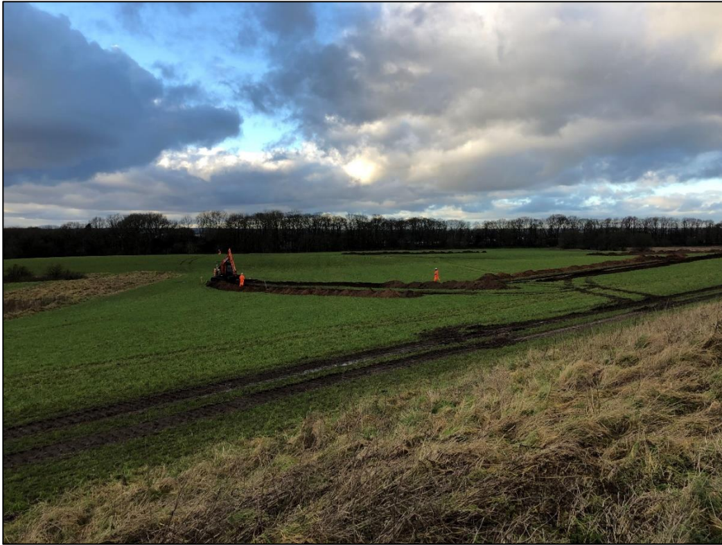
Plate 1: General view over southern section of Area1, trenches 143, 135, 136, 138
