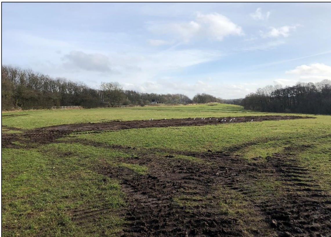
Plate 15: General view over Area 4 after backfilling Trench 026-031
